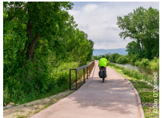
Wilson to Namaqua Trail paving
